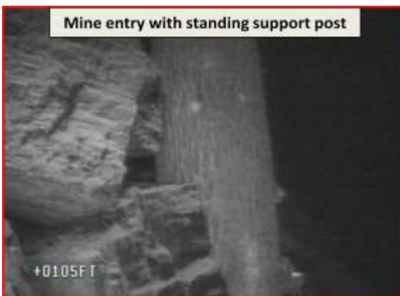
Open mine entry with intact roof rock
